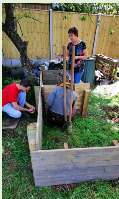
Constructing the composter
